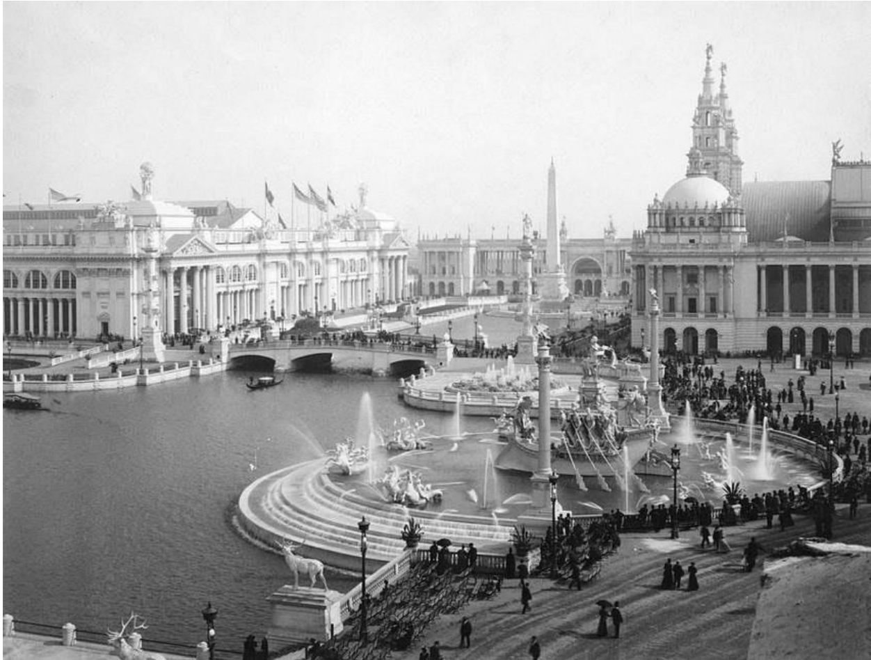
A few of the 200 mostly temporary buildings at the 690-acre 1893 Chicago World's Fair which was built in 3 years.
