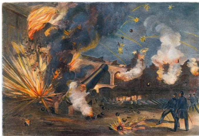
THE DESTRUCTION OF FORT SUMTER BY THE BOMBARDMENT
